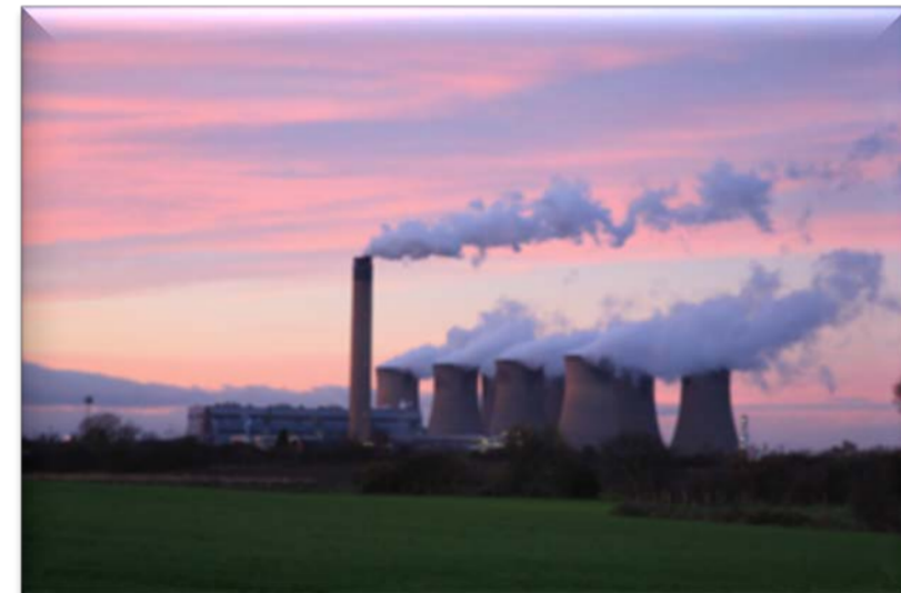
Drax power station
